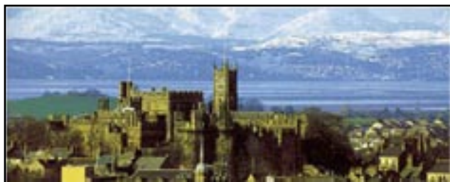
View of Lancaster
