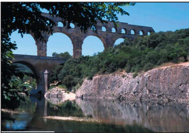
Pont du Gard, south France - one of the photographs in the Image Bank. Image donated by Kim Biddulph, Buckinghamshire County Council
